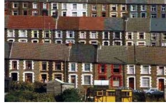
Terraced houses are joined to other houses on both sides .
